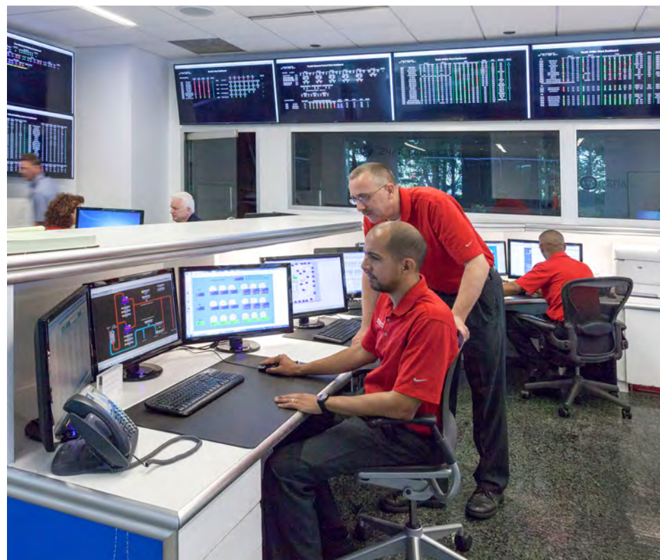
JBG SMITH TENANT SERVICE CENTER, NATIONAL LANDING
